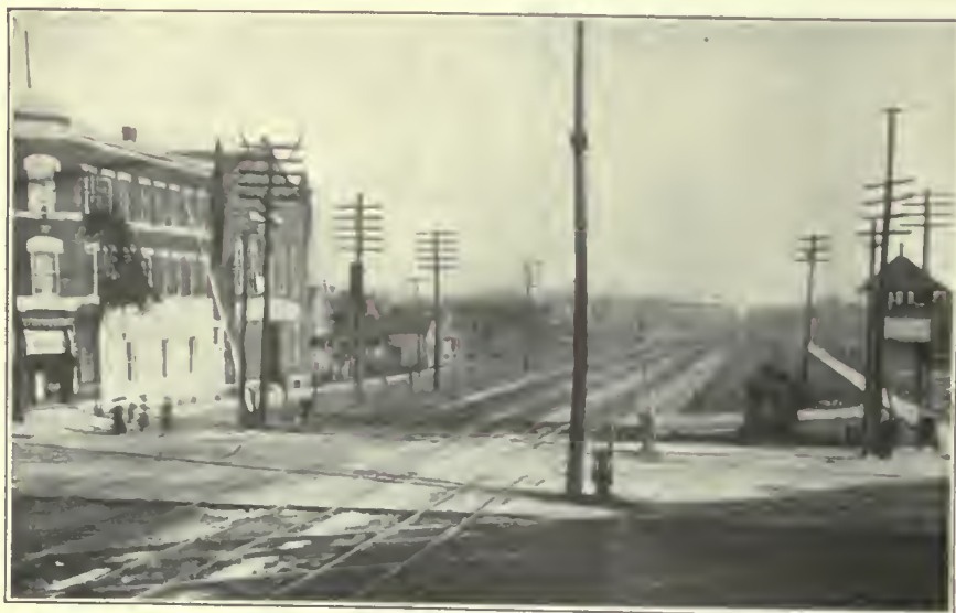
FIG. 254. GRADE CROSSINGS. Hammond, Ind., crossings of the Michigan Central Railroad, the Chicago & Erie Railroad and the New York, Chicago & St. Louis Railroad.
